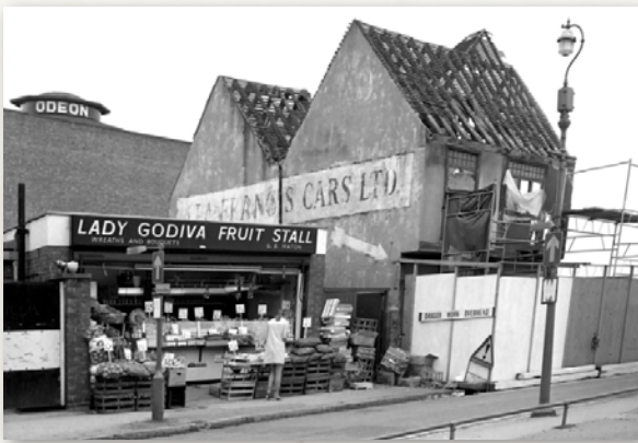
No 7 Much Park Street just before demolition in the late 1960s. Nos 8-10 had just gone, along with 11-16 and the Gloria Works. Everything to the left had been destroyed in the Coventry Blitz of 1940 but Lady Godiva made the best of it. The interesting thing about this photo is that Lea Francis have arrowed the direction to their factory – which was the old Triumph one.
