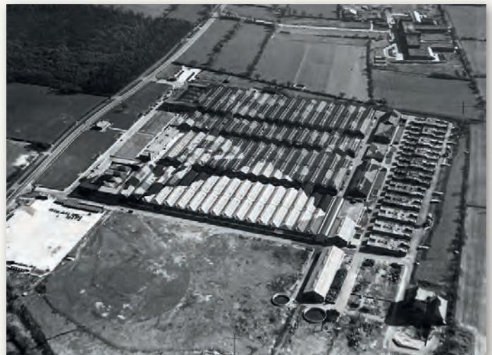
The Shadow Factory built on Banner Lane in wartime camouflage. Banner Lane itself is on the left and the ten silos at the rear of the buildings were aero engine test cells.
