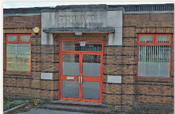
'Triumph' is still showing over the front door of what is now 'Tenable House' on Torrington Avenue. This was the building put up by ACMC in which to manufacture Triumph bicycles after the war. By then the two concerns had separated and been moved away from Central Coventry. But both ended up under a mile away from each other.
