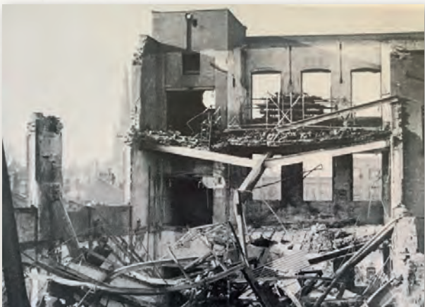
An area of the Priory Street factory, on the morning of 15th November 1940.
