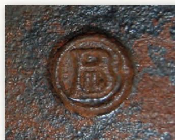
The Beans Industries Limited mark cast into a Stag block. You can just see the 'IL' inside the bottom of the 'B'.
